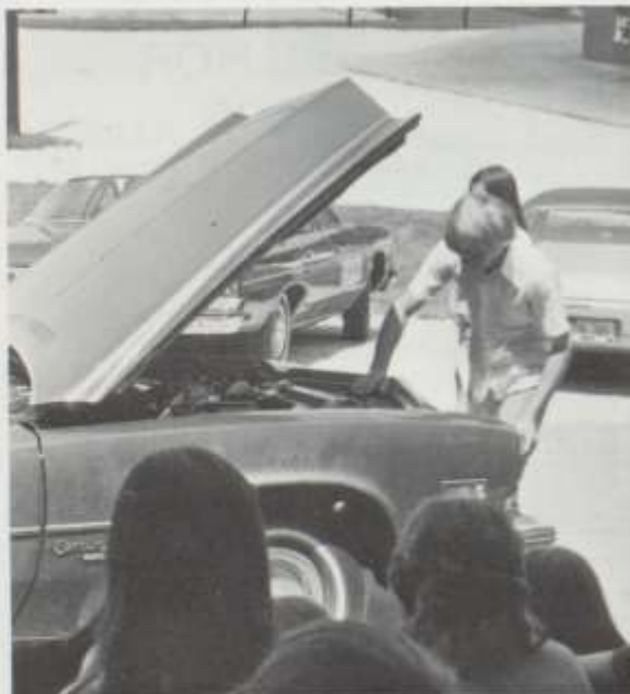
George Eichmiller demonstrates to the driver's ed class the proper procedure for checking the water level in a radiator.
